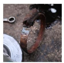
Clip is cut with a grinder & removed.
