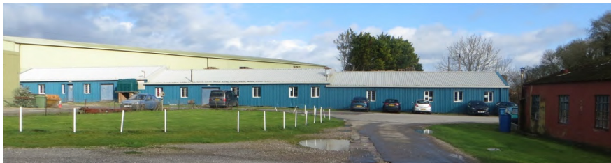
The blue building is the old Thruxton Race Shop, reception on the right, assembly on the left.
